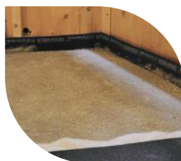
Laying of acoustic mats
